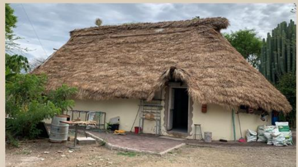
The new dining room's roof
